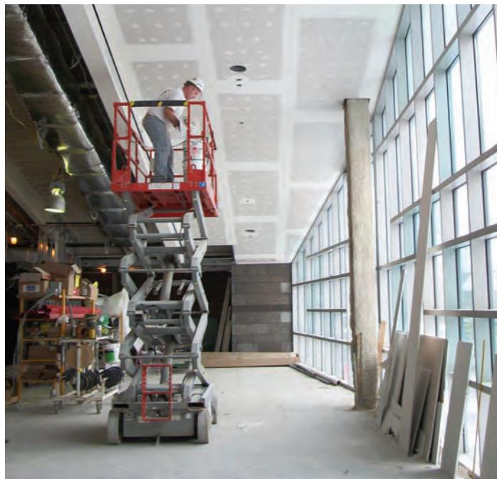
The extensive use of natural light creates a soothing environment and is eco-friendly.
